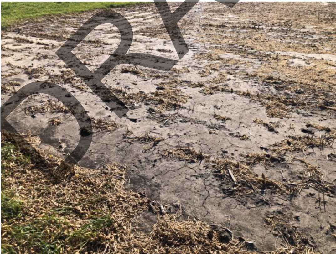
Photo 14 – surface soil crack at edge of field
