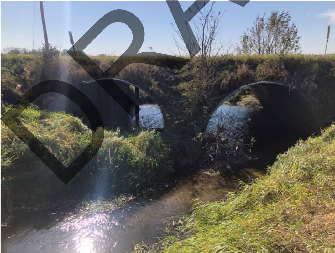
Photo 10 – SE 18 th St bridge over unnamed stream, looking southwest
