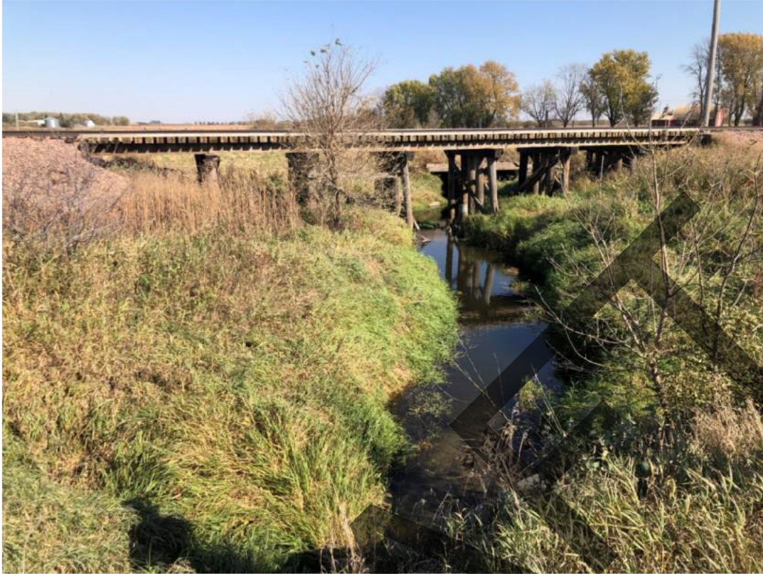
Photo 9 - Railway bridge over Unnamed stream, looking north
